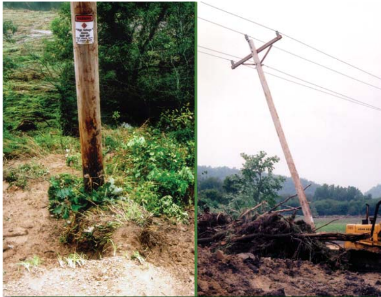
Typical pole damage caused by flooding included ground washed away around the base of the pole (pictured at left) and debris carried by floodwater left pushing up against a pole (right).
