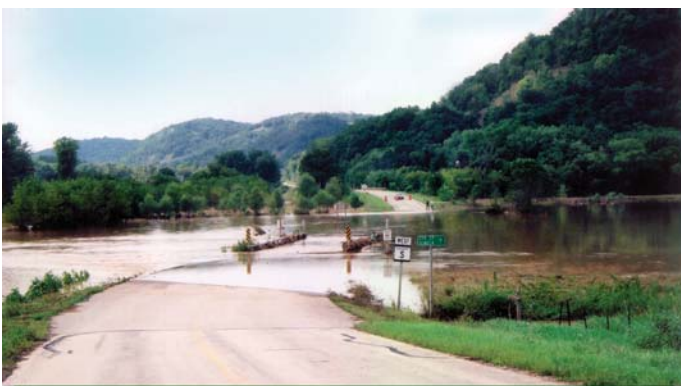
Washed-out bridges and flooded crossways like this divided SREC’s Crawford County service territory and presented accessibility problems for days after the water receded.
