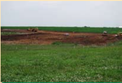
Darlington: Site preparation and street infrastructure are being worked on.
